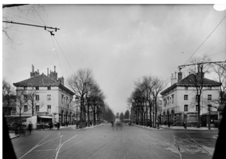
24. Facade and perspective view towards the statue of the Lion of Belfort. 3 - 4 Avenue du colonel Henri Rol-Tanguy, Place Denfert-Rochereau. Paris 14. . Photograph by Edouard Desprez. © Edouard Desprez / DHAAP / Roger-Viollet
